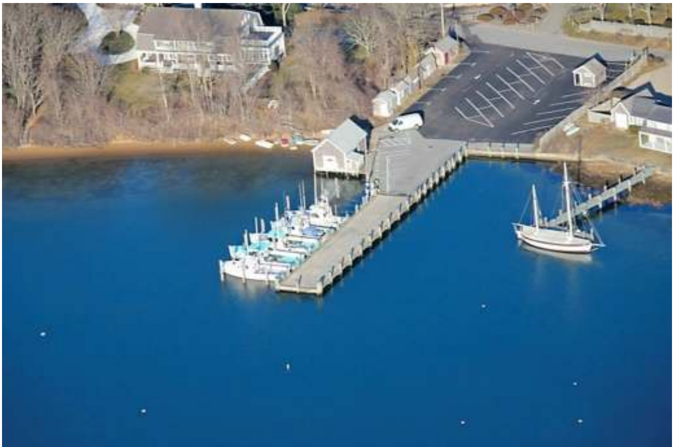
Figure 2. Aerial picture of the site after the project was completed; the new system is entirely underground. (courtesy Tom Leach)
